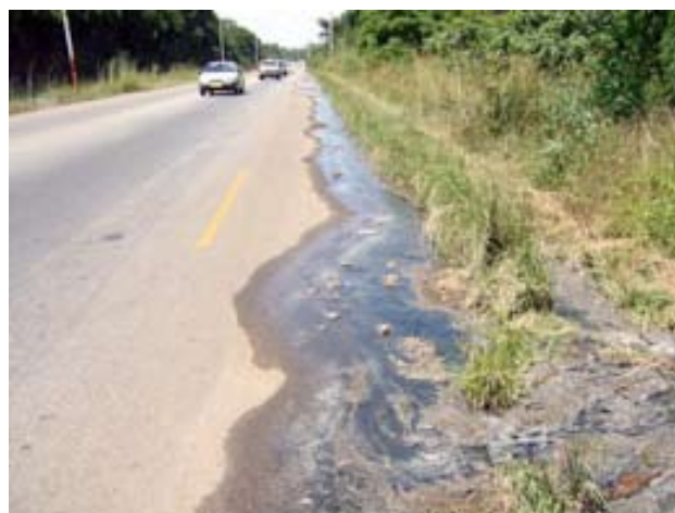
Figure 12. Effluent from breached sewer
